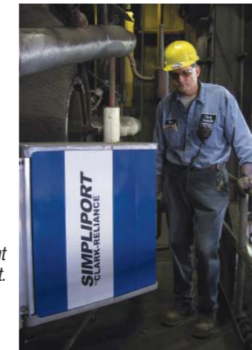
100 year old power plant with Simpliport retrofit.
