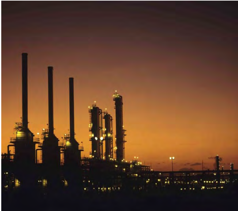
Figure 1. For certain industries, a DCS provide substantially more value as the basis for automating the plant than a PLC-based system.
