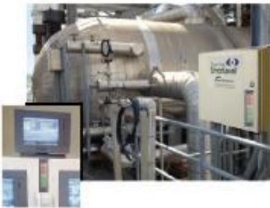
Eye-Hye® SmartLevel™ Local and Remote Indicators
