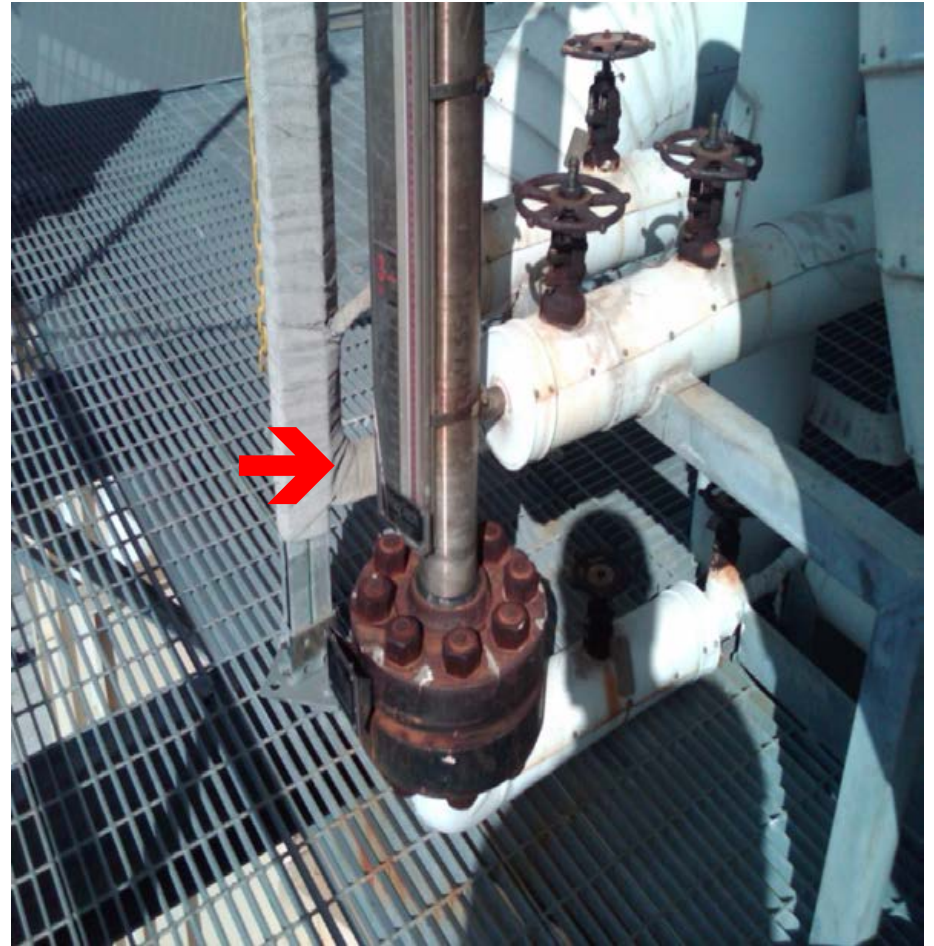
Magnetic Level Gage Scale extends below lower connection, it will always indicate some level
