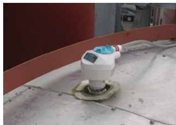
The compact SITRANS LR250 can be installed in small vessel openings and close to the vessel walls.
