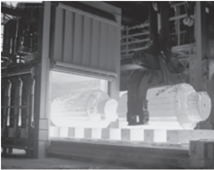
Butterfly valve BVHM on forging furnace to reduce the oxygen level
