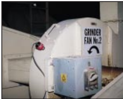
Broken Filter Bag Detection
